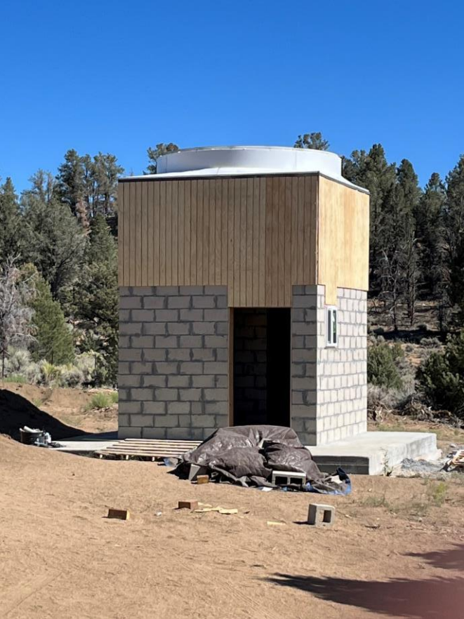
Fiberglass Skirt and Dome Ring Installed
