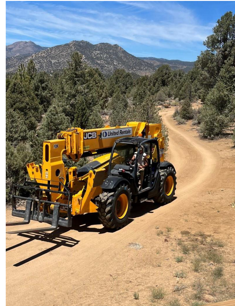
Martin and the Crane “On-Site”
