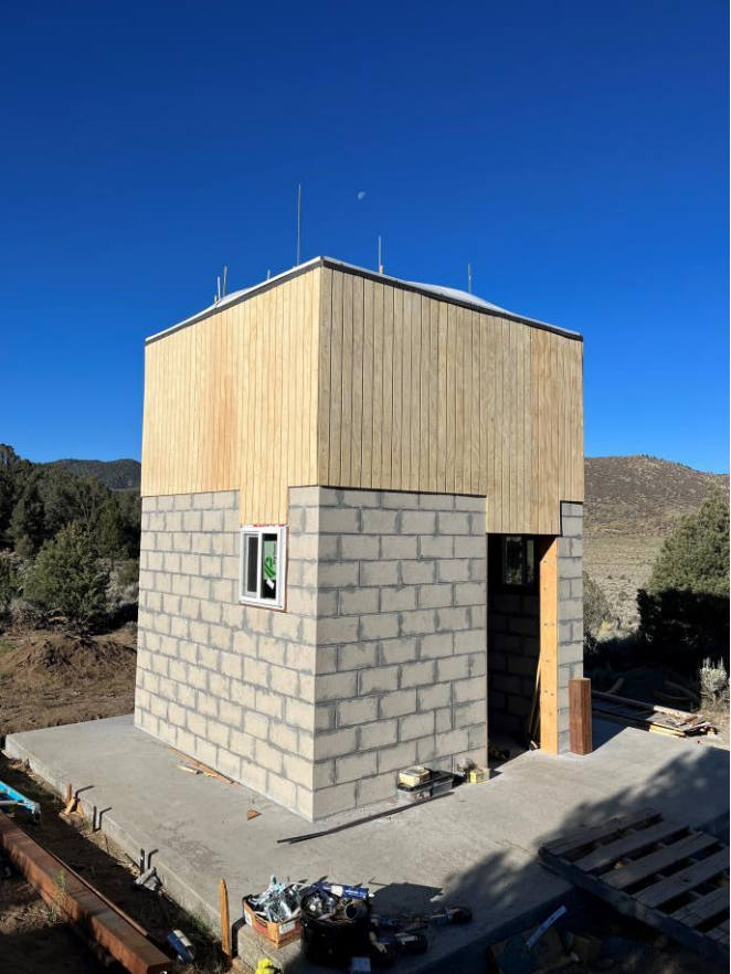
T-111 Siding install complete
